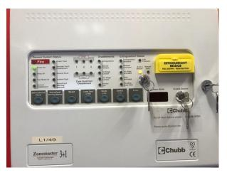
A Sigma XT control panel sits outside the IT computer room and lights flash to show any identified faults. This control panel monitors the environment within the room.
